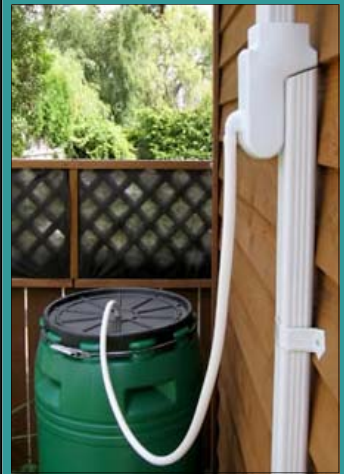
"CLOSED-TOP" BARREL WITH DOWNSPOUT DIVERTER
