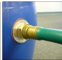
Both ends of the connective hose can then be screwed into the linking ports.
