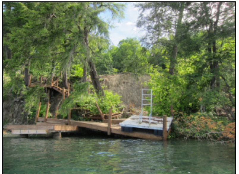
Lakeview of improperly sited camp road causing erosion along the lakeshore.
