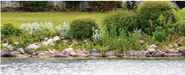
**Vegetated Rip-Rap**—The stones prevent erosion along the shoreline from wave action while the vegetation roots into the soil, binding it into place.
